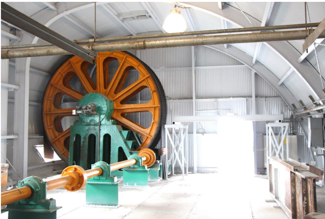
Condition Photo 10: Inside machinery enclosure on west tower.
