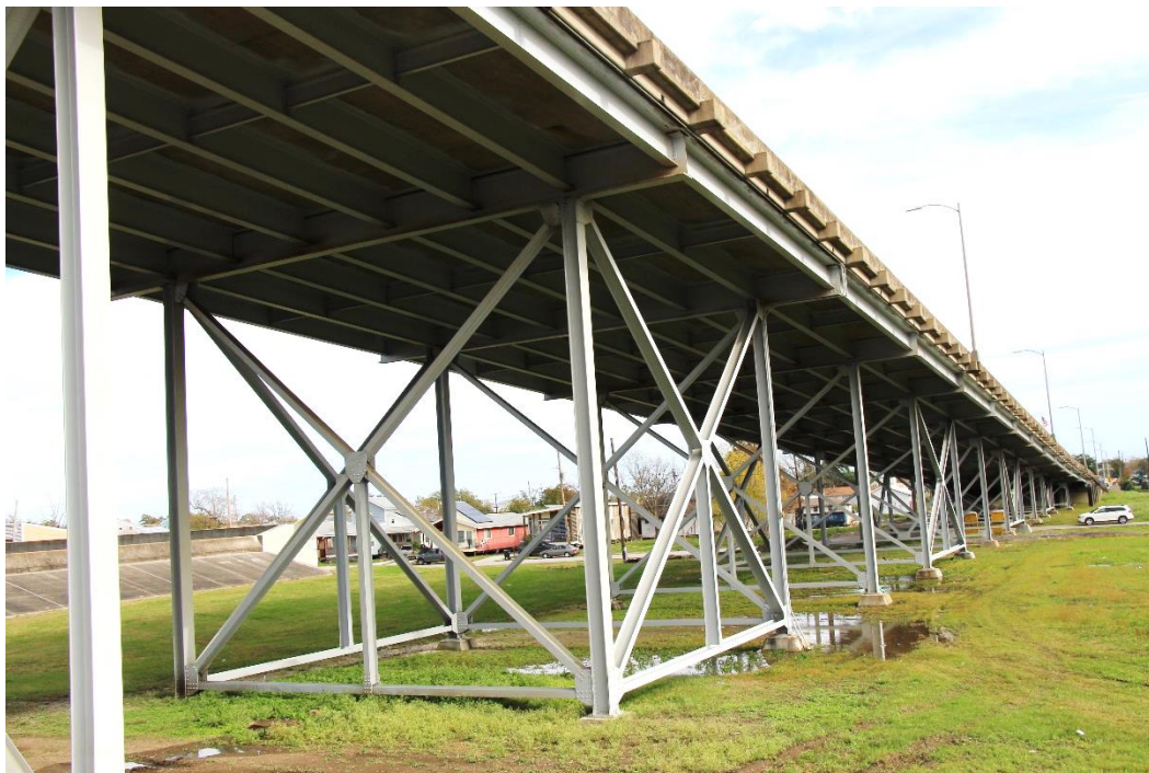
Condition Photo 16: Easterly approach spans superstructure and bents.
