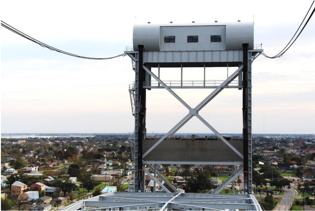
Condition Photo 7: East tower machinery enclosure (west tower is similar).
