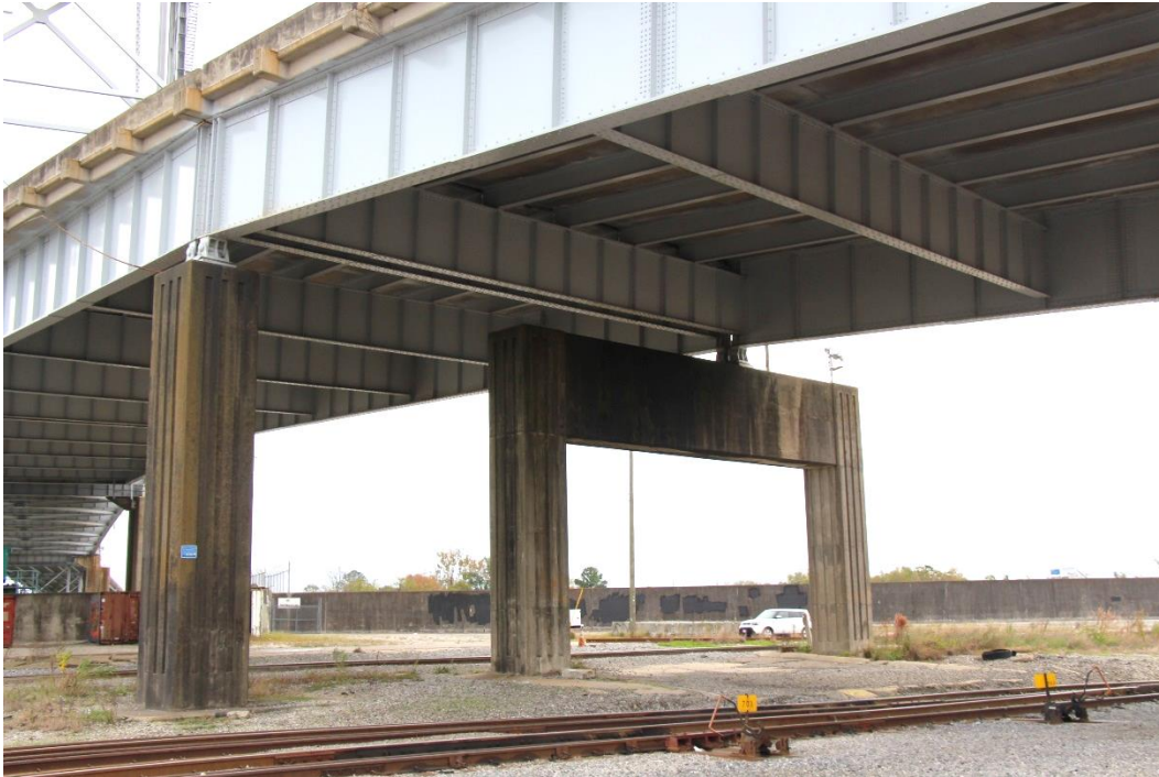
Condition Photo 13: Westerly approach spans superstructure and substructure, looking northwest.
