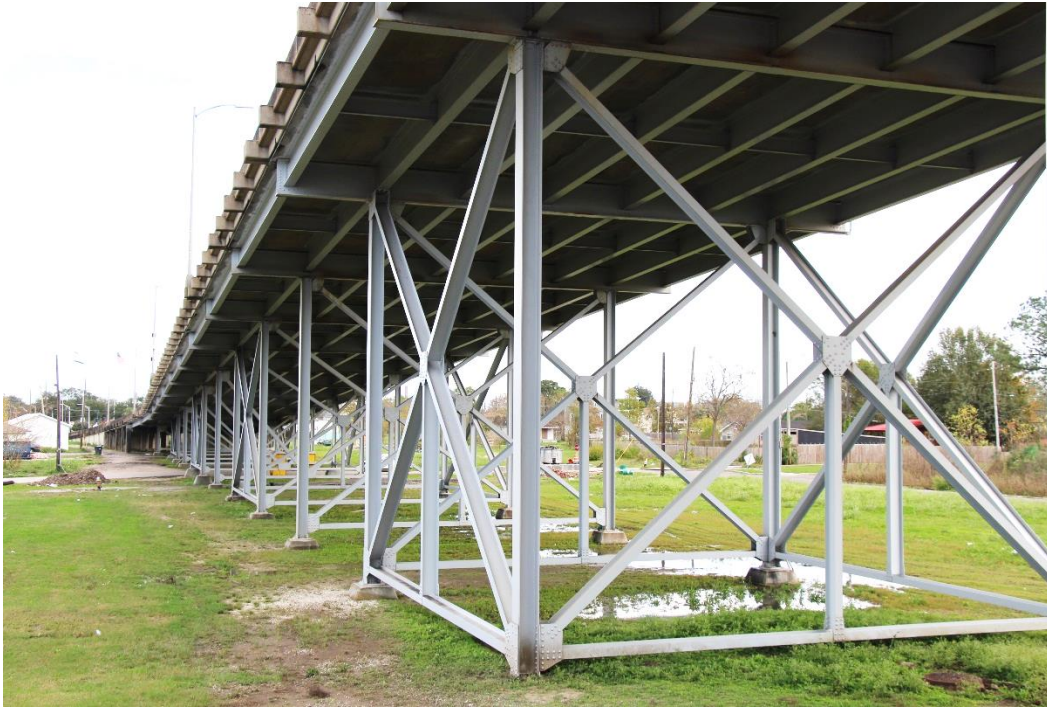
Condition Photo 17: Easterly approach spans superstructure and bents.
