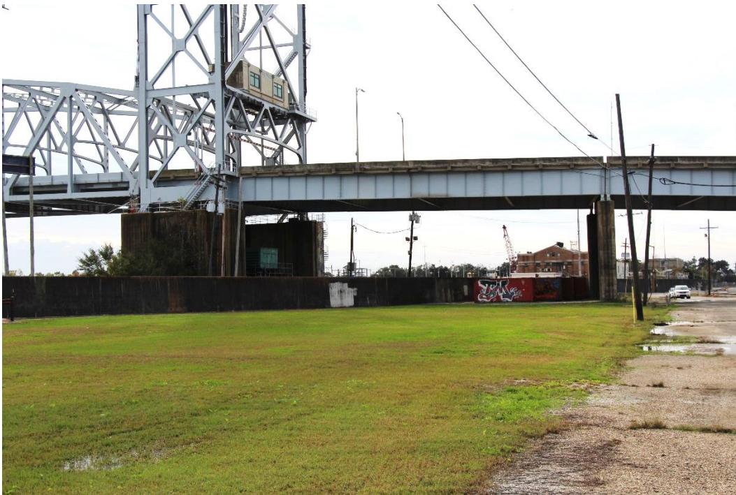
Historic Fabric Photo 1: Steel plate girder approach span on west approach to vertical lift span.
