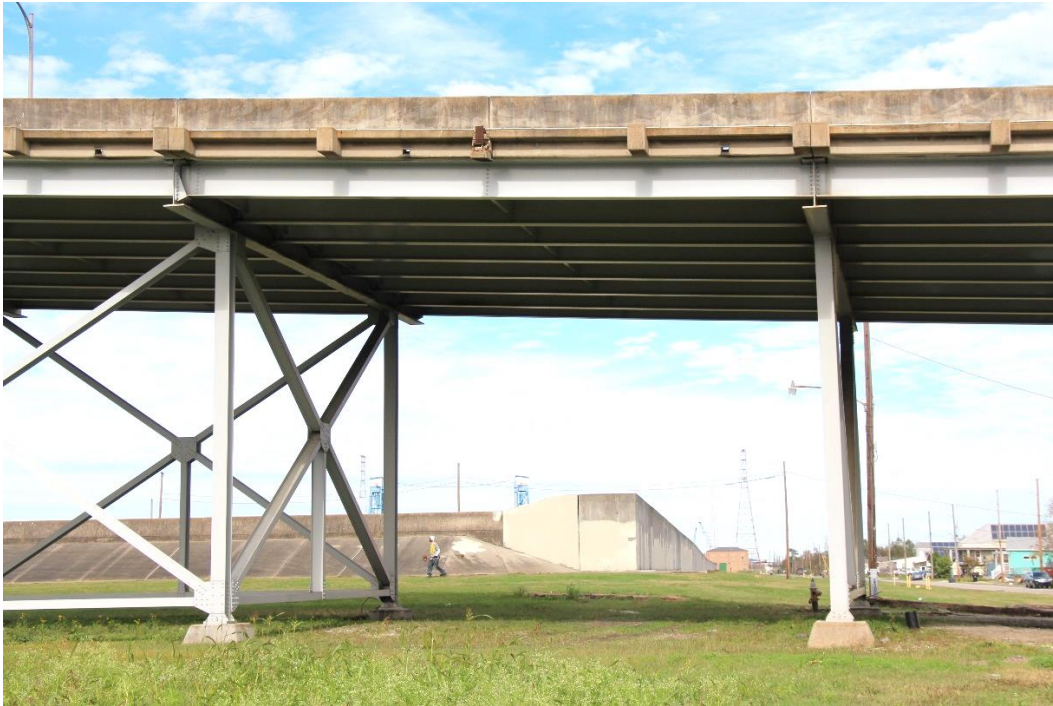
Historic Fabric Photo 2: Typical steel beam approach span and substructure.
