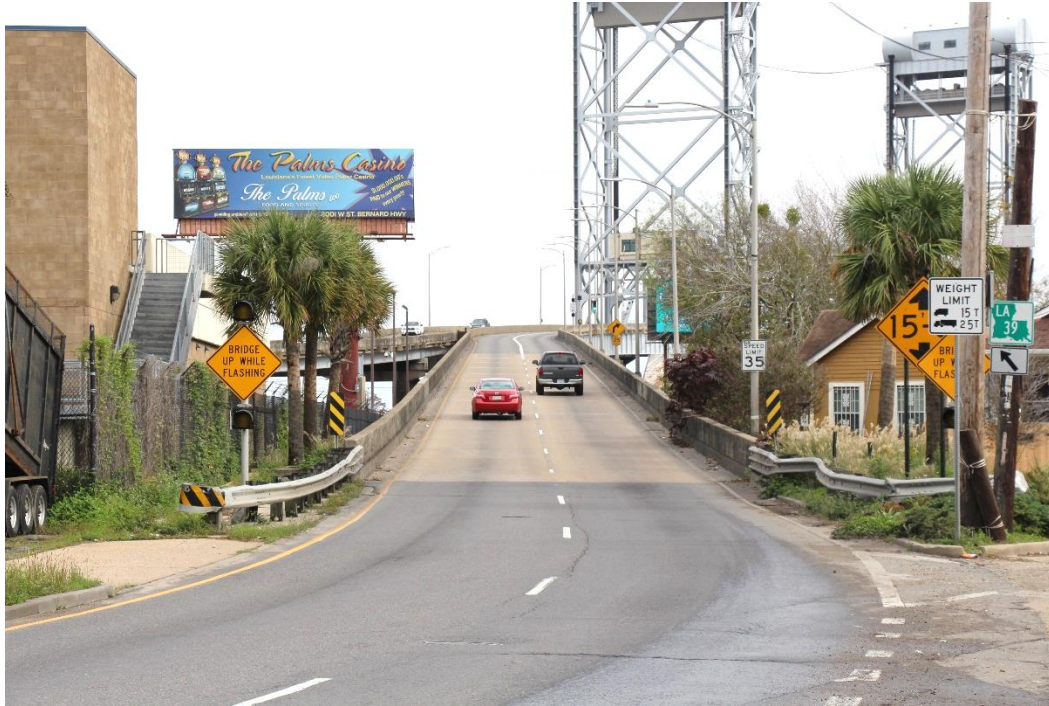
Condition Photo 15: Westerly approach spans of Recall No. 001610, leading up to Recall No. 020375 (Judge Seeber Bridge), looking east.
