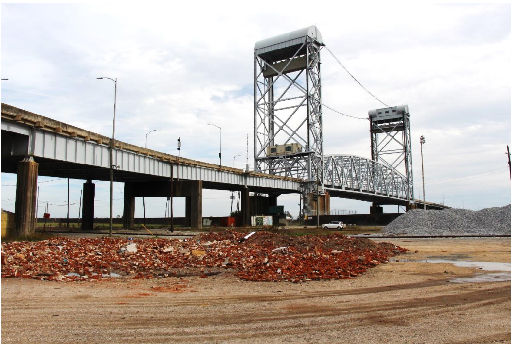
Condition Photo 14: Westerly approach spans overview, looking east.
