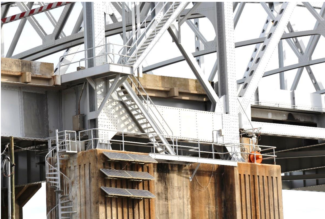
Condition Photo 2: West tower span, stairs, platforms, and pier.
