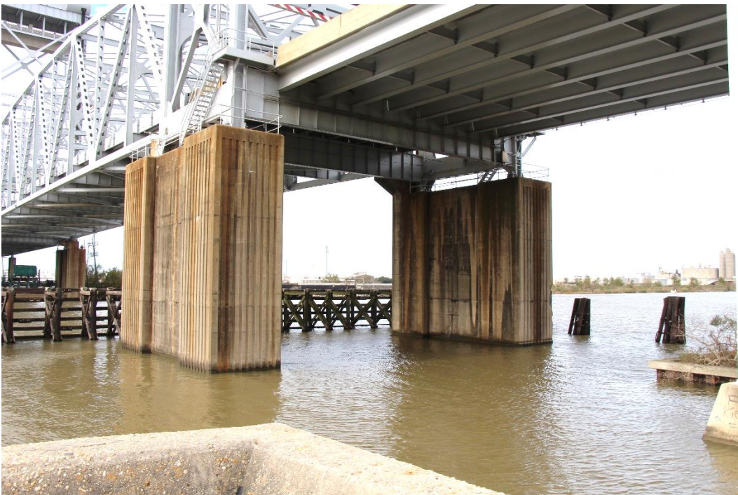
Historic Fabric Photo 3: Concrete main-span substructure.
