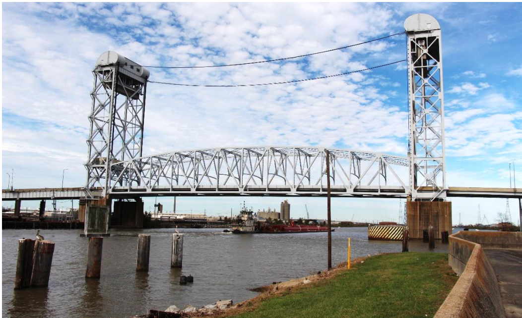
Character-defining Feature Photo 1: Design and construction of a vertical lift span with lift-tower drive machinery. A set of motor and drive machinery is located at the top of each lift tower. Each machinery set drives two sheaves to raise and lower the lift span.
